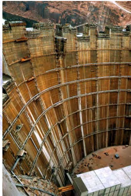
(dam construction, 1963 explorepdx.com)
