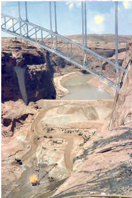
(coffer dam during construction, 1959 explorepdx.com)
