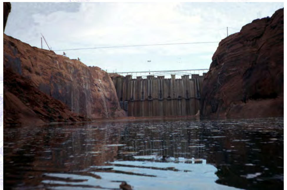
(back of Glen Canyon Dam during construction, 1963 explorepdx.com)
